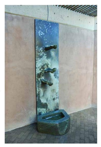
through a gutter into a 50-gallon tank, then through copper tubing into the first of the cast bronze hands, pouring over the other two arms and into the stone basin. The overflow then streams toward the drain in the middle of the patio. If the roof tank fills to capacity, the water will take approximately thirty hours to flow through the fountain.
